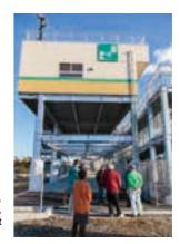
This tsunami evacuation tower, completed in 2016, makes it possible to evacuate to levels above 6 meters, which is high enough in relation to the estimated height of inundation.
