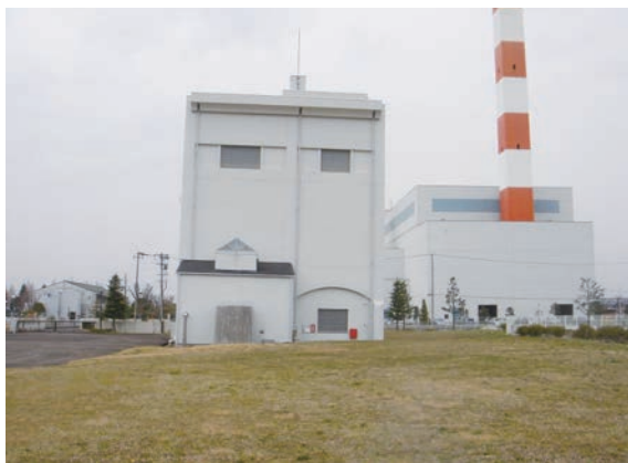
The Imaizumi Pumping Station tilted by the earthquake
