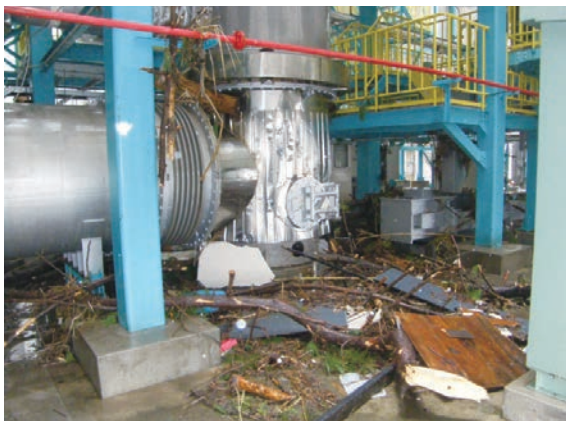
Damaged incinerator
