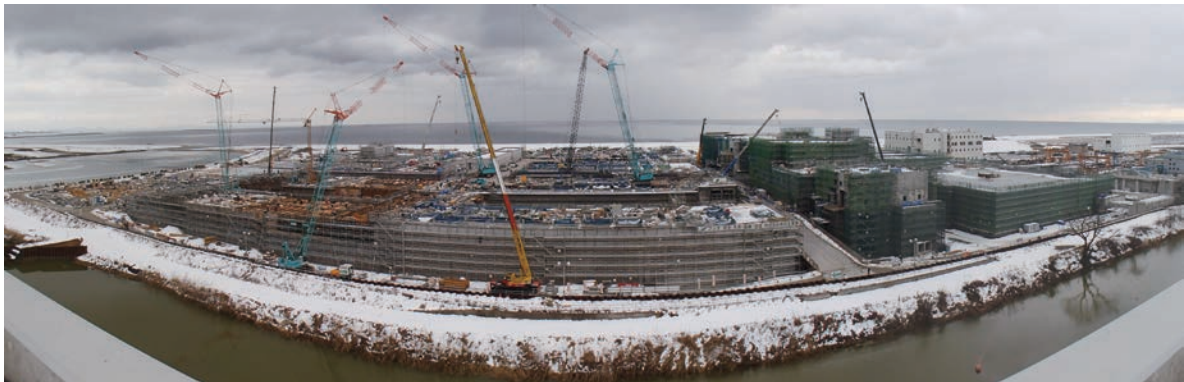
Minami-Gamo Wastewater Treatment Plant (Feb. 3, 2015)
